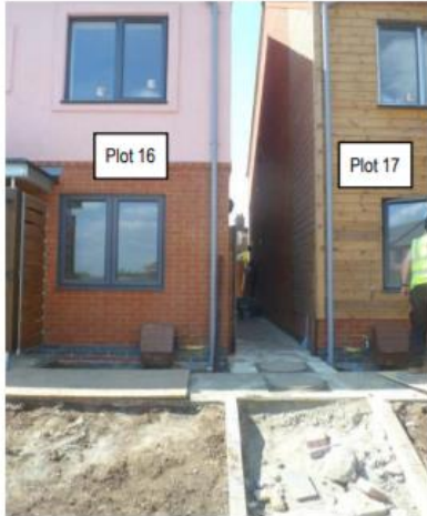
Plot 16 Soft Landscaping Formation Pre Topsoil Placement
