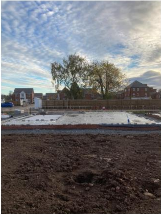
Plot 94 – Location of Hand Excavated Trial Pit
