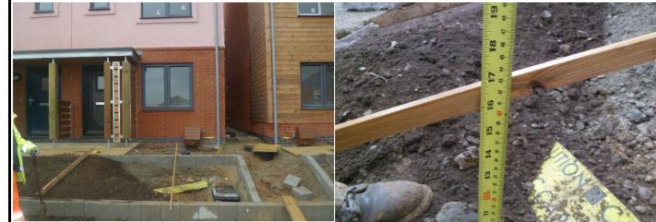
Soft Landscaping Area Adjacent to Road - In Front of Plots 15/16
