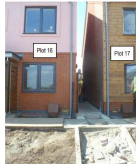
Plot 16 Soft Landscaping Formation Pre Topsoil Placement
