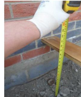
Plot 16 Soft Landscaping Formation Pre Topsoil Placement
