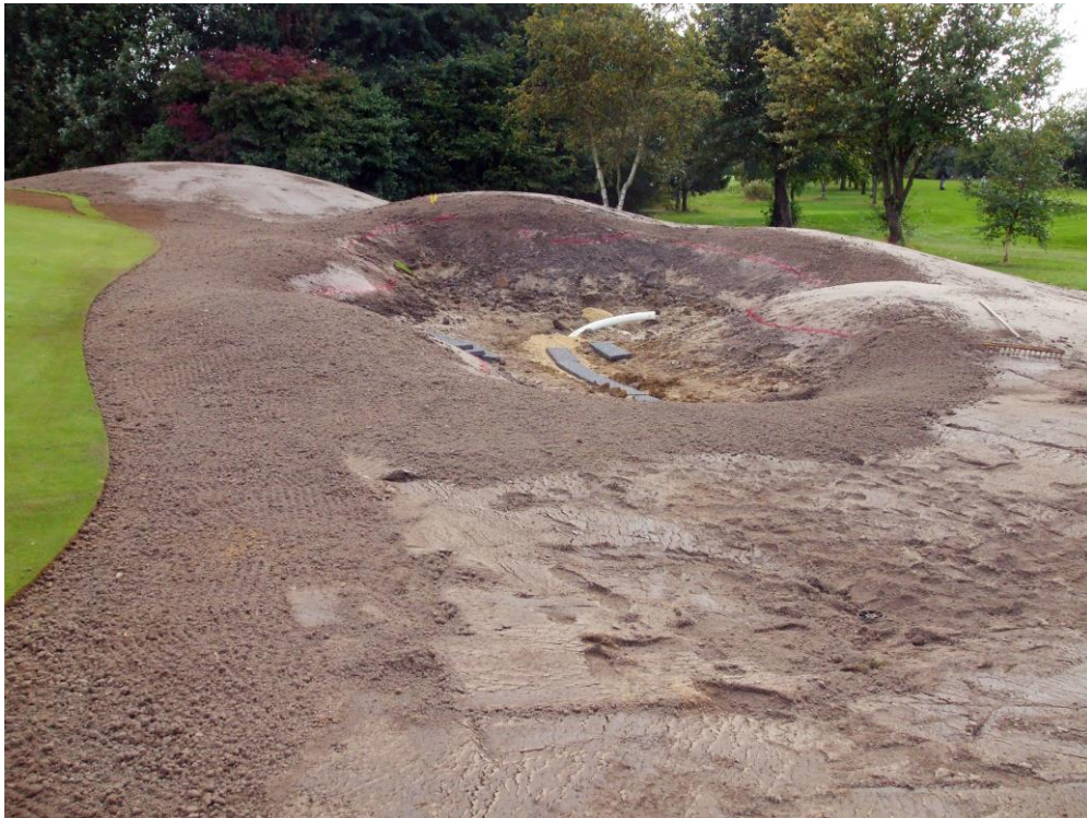
Forming the bunker with Landscape20.
