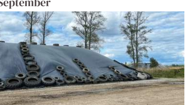
Completed the building and sheeting of outside stocks to ensure supply is maintained
